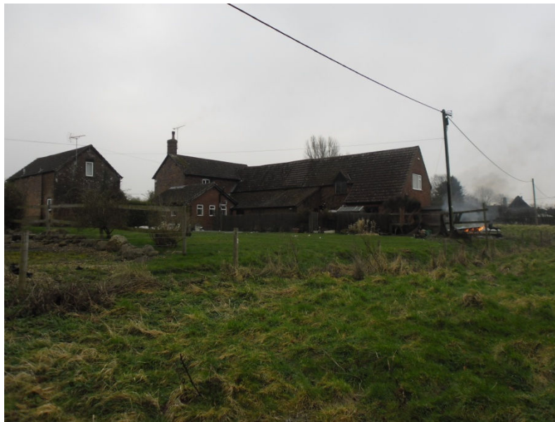
Plate 8: Rear elevation of public house and outbuilding
